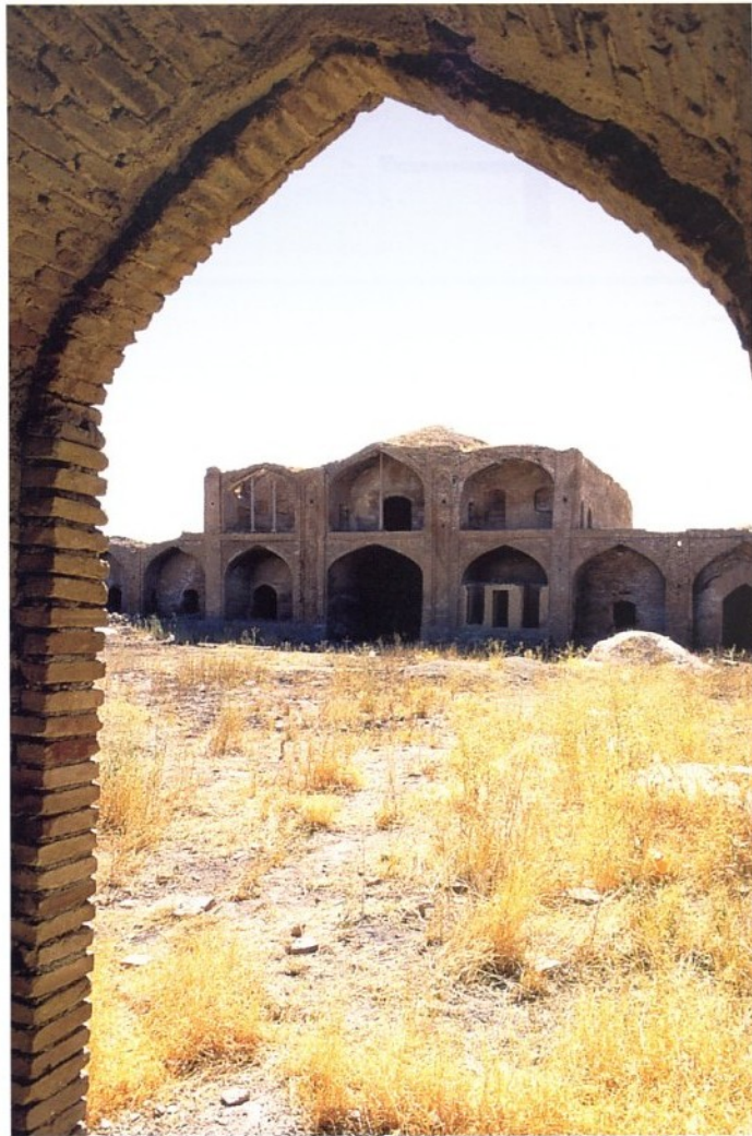
95. Entrance portico from inside the courtyard
