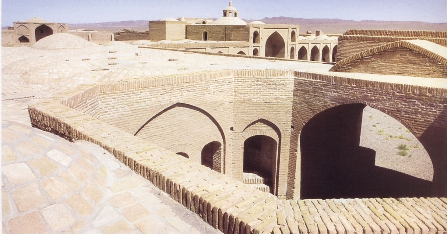
66. Courtyard behind the southwestern eivan of the eastern courtyard
