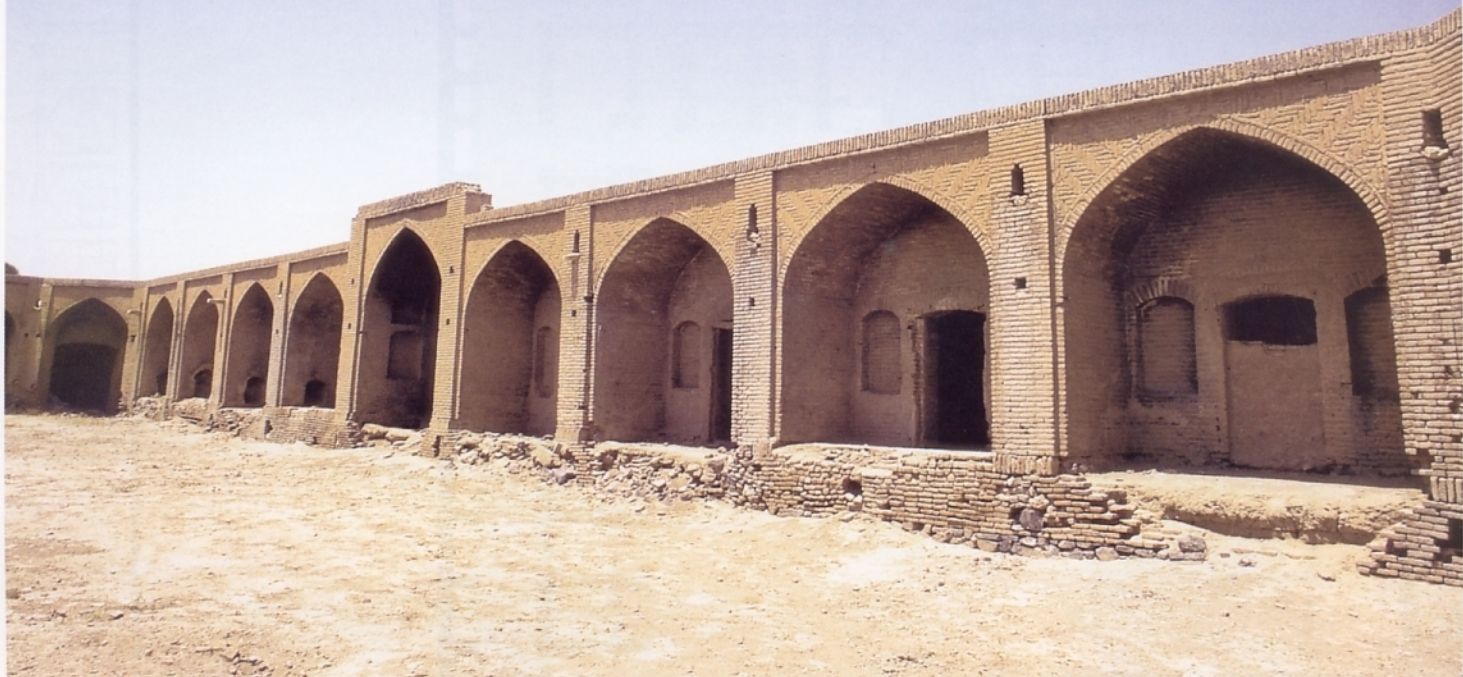
29. Southern courtyard, eastern side
